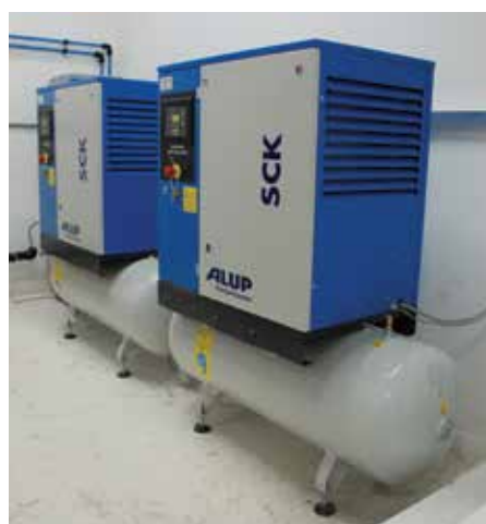
Two compressors on buffer vessels
