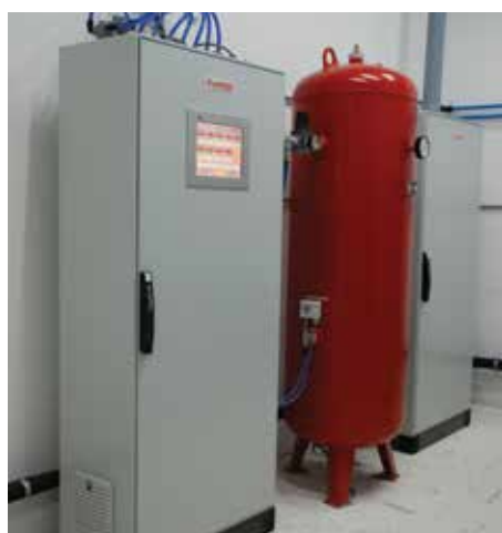
Two standing cabinets for generator and distribution system with inbuilt control unit and separate hypoxic air buffer vessel
